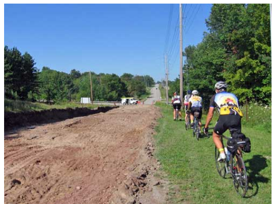
First road construction
